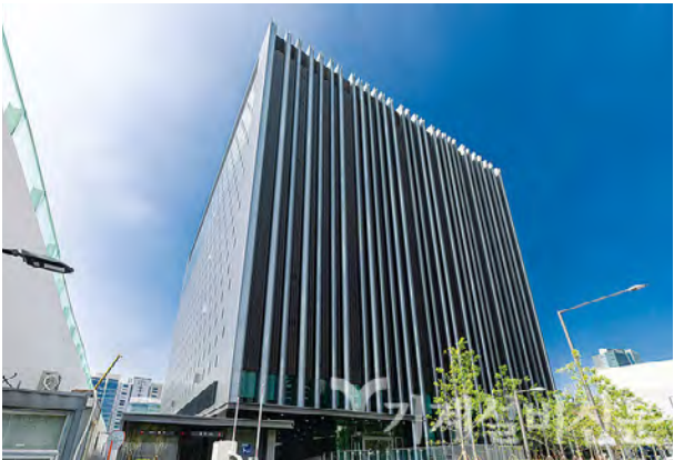
Gasan Center, the largest in Seoul
